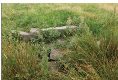
Plate 43 - Culvert in centre of Field 17
