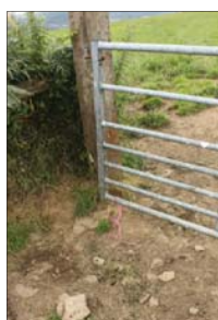
Plate 58 - Close up of gate to Field 39 in disrepair
