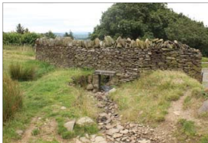
Plate 41 - Culvert through wall in south-eastern corner of Field 9
